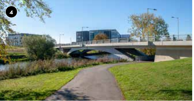
Northampton Waterside Bridge
