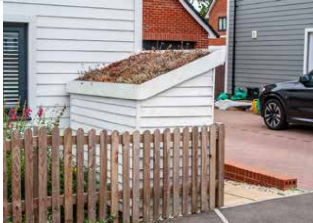
Green roofs on bin shelters to help capture rainfall whilst making a more visually appealing street (Arborfield Garden Village, Berkshire).
