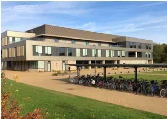
Covered, cycle parking that is located close to the building entrance (Trumpington Meadows, Cambridge).
