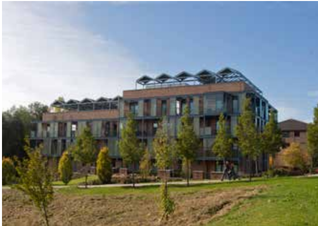
Solar panels on roof orientated to capture maximum sun exposure create an interesting architectural feature on the building (Campbell Square, Milton Keynes).
