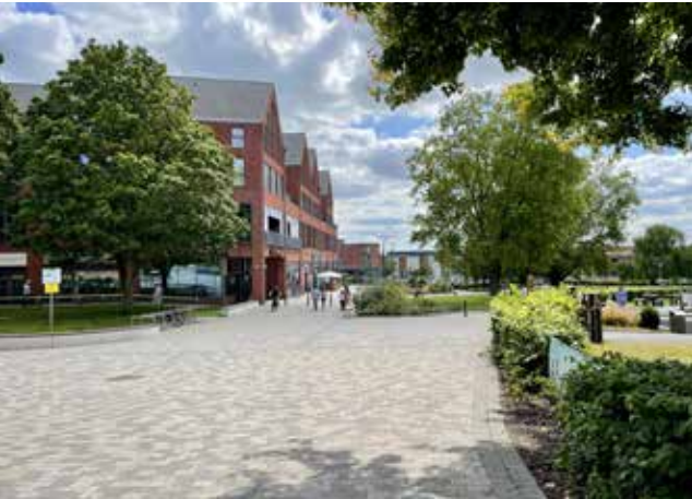
Active, ground-floor retail units, framed by formal landscaping and a flexible, public realm space that can support a range of activities (Elms Field, Wokingham).
