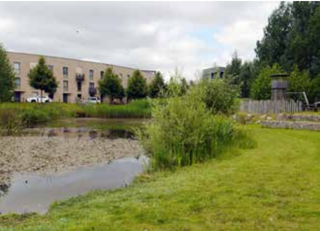
Green buffer around SuDs basin to manage any overflow during periods of heavy rainfall (Barton Park, Oxford).
