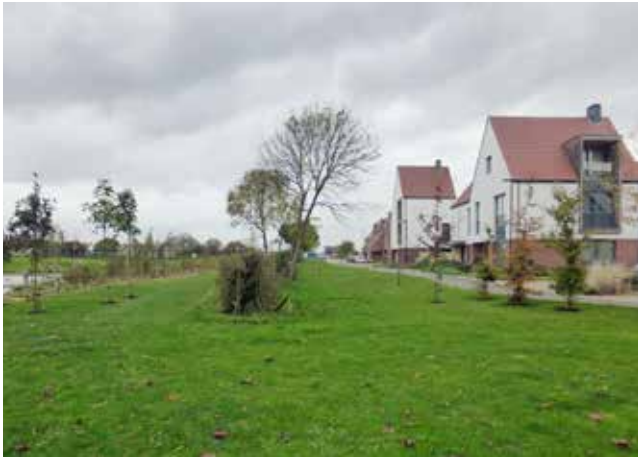
Buildings with a lower height look out to the landscaped space with frequent tree planting that helps to break up the feel of a continuous built frontage (Derwenthorpe, York).
