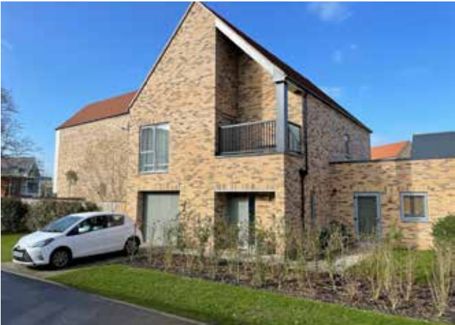
On-plot parking designed to have minimal visual impact along the building frontage, sitting within front garden planting with a smaller, garage door that uses the same material palette as the rest of the house (Beaulieu Park, Chelmsford).
