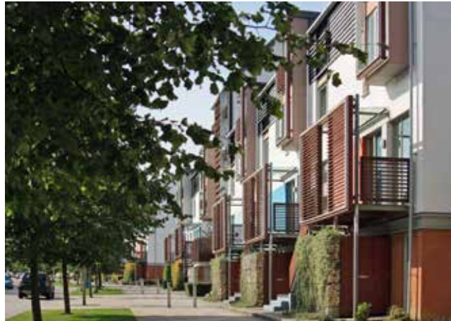
Large brise-soleil system, combined with manually operated shutters prevents overheating in the summer months (Newhall, Harlow).
