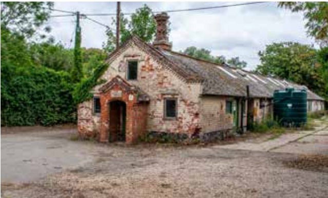
Existing brick buildings with detailing around the doorway and chimney to be celebrated as a heritage asset.
