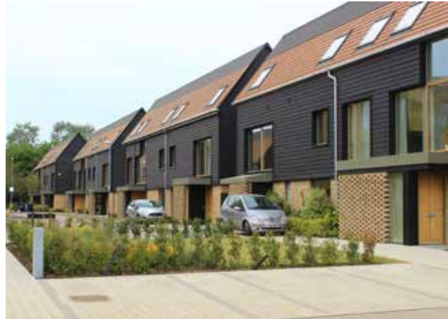
Gutters and down pipes along the building frontage help capture rainwater and channel it to either water butts or rain gardens on individual plots. (Great Kneighton, Cambridge.)
