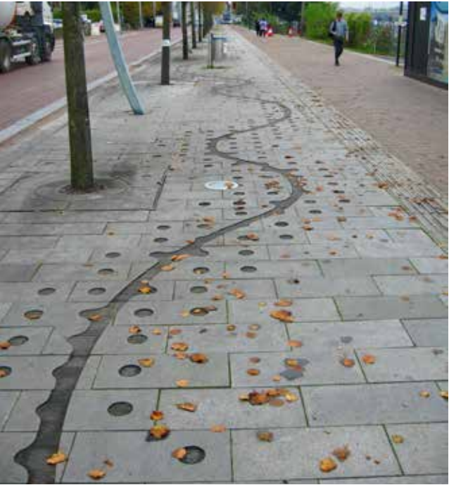
Attractive permeable paving that helps to naturally manage surface water and support healthier landscapes (Utrecht).
