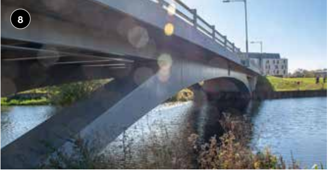
Northampton Waterside Bridge
