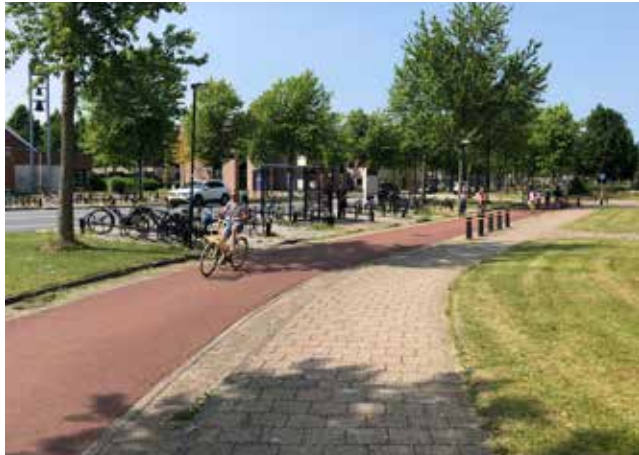
Segregated cycle route separated by a generous green verge to vehicular movement, successfully creates a safe, uninterrupted active travel link (Houten, Utrecht).
