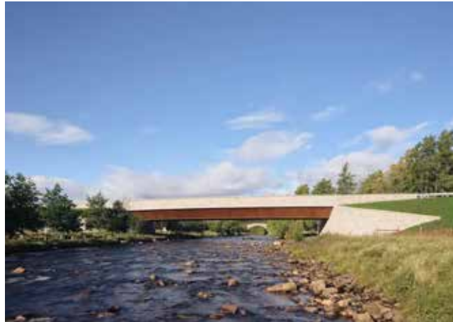
A bridge that forms a bold architectural statement, elegantly spanning the valley and embracing the surrounding landscape while enhancing its natural character (Gairnshiel Jubilee Bridge, Scotland @Moxton Architects).
