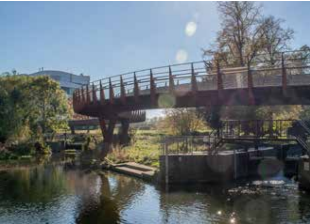
Bridge that support active travel movement to ensure people can cross even during heavy rainfall or flooding (Northampton).
