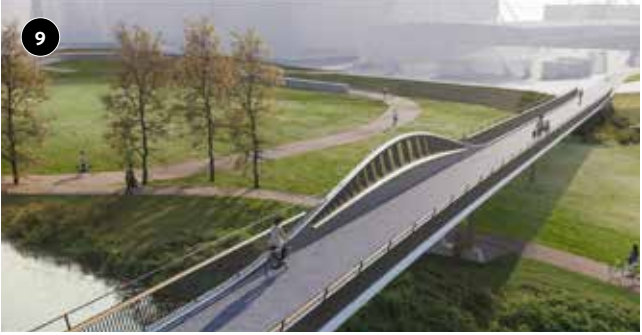
Oxpens River Bridge (Oxford)
