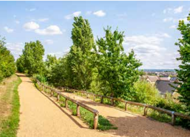
Multifunctional acoustic barrier that not only minimises noise from the adjacent motorway but also supports a gentle ramp up and along it to create a new leisure route (Milton Keynes).
