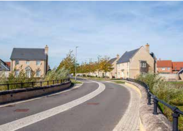
The configuration of the bridge, framed by soft landscaping and well-proportioned homes, creates a welcoming transition and a subtle gateway into the new development (Alconbury Weald).
