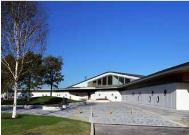
Shared surface space with street furniture prioritises active travel movement to school. (Alconbury Weald Primary School).
