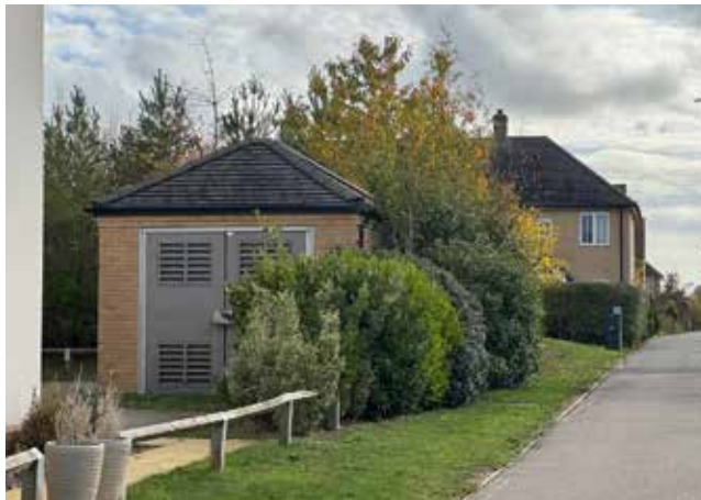
Substation integrated into urban fabric (Alconbury Weald).
