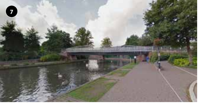
Wharf Road Bridge, Newbury (@Google)
